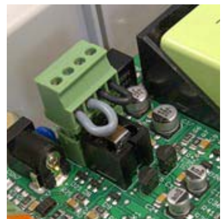
Fig.: cable bridge
