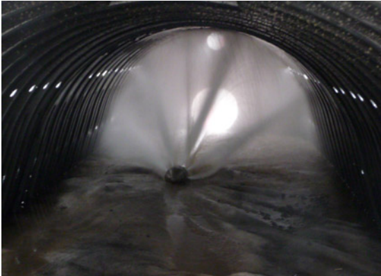
Image 4: Flushing nozzle with cleaning procedure
