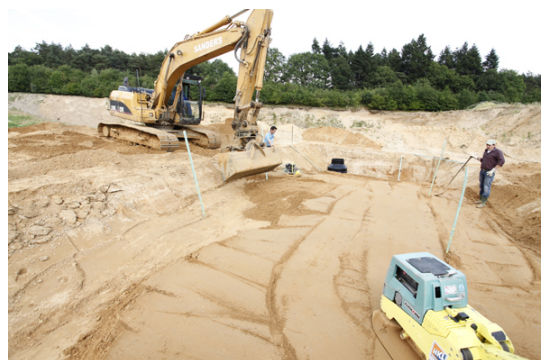
Image 13: Covering the tunnel elements
