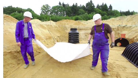
Image 7: Woven filter fabric on bottom area
