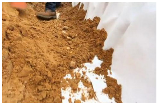
Image 11: Backfilling filter fabric for fixing
