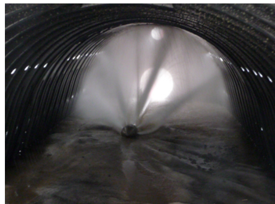
Image 15: High pressure cleaning
