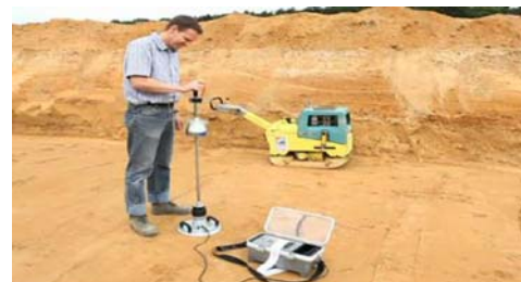
Image 6: dyn. Plate load test at ground level
