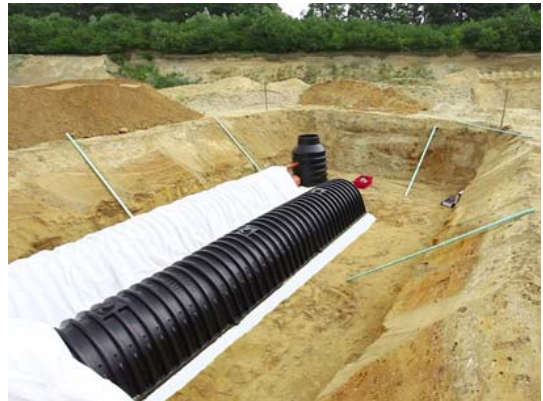
Image 10: Covering with filter fabric
