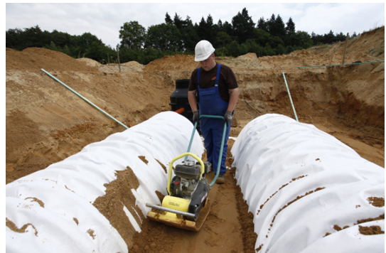
Image 12: Compacting with a small compacting device between rows of tunnel
